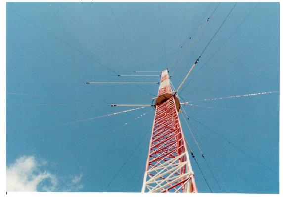
Full sized 1/4 wave elevated feed vertical. Tower is 18" face Pirod with base insulator at 60 feet. There are 24 elevated radials.
