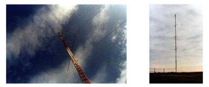
4/4/4/4 modified/extended HyGain 155BA' for 15 meters on a 180 foot tower. Tower is 18" face Windcharger. Each ant is independently steerable.
