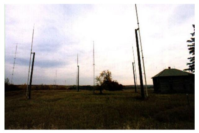
One of the primary 80 meter antennas is a switchable 4 element vertical beam, switchable NE NW SE SW, it consists of a center feed point and 4 parasitic elements that can be electrical changed to become
