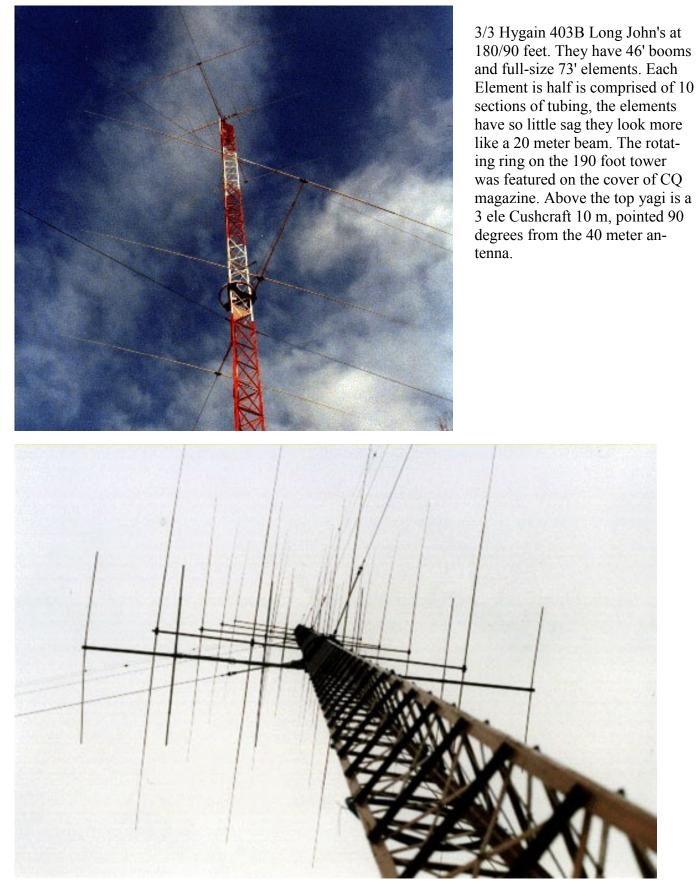
This spot is looking straight up the 20 meter rotating tower. 4/4/4/4 Hygain 204BA's the rotatable towers Paul uses a trim motor from a B27 to rotate the tower.
